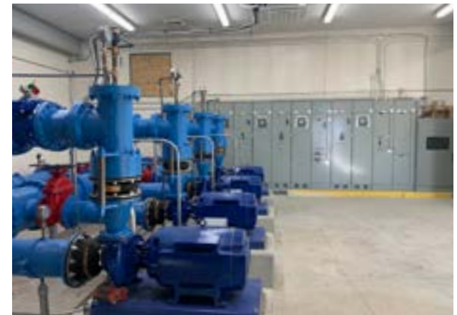
Rosecrest water pump station upgrade
